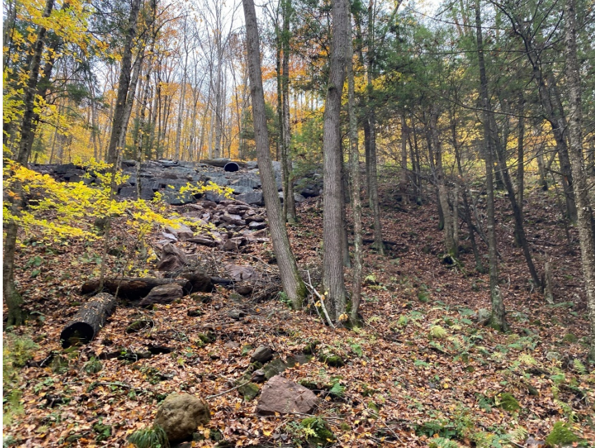
Image 4: View of rockery wall from down-slope at Site 1 at Worlds End State Park
