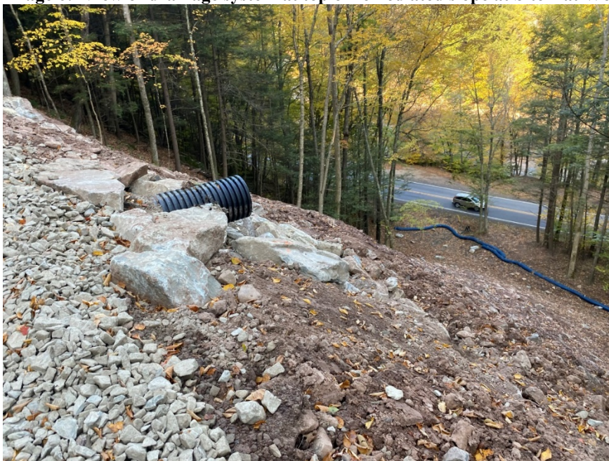
Image 6: View of drainage system at top of remediated slope at Site 2 at Worlds End State Park
